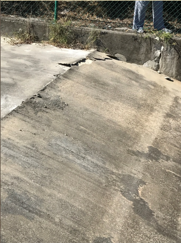
Cracks in cement
